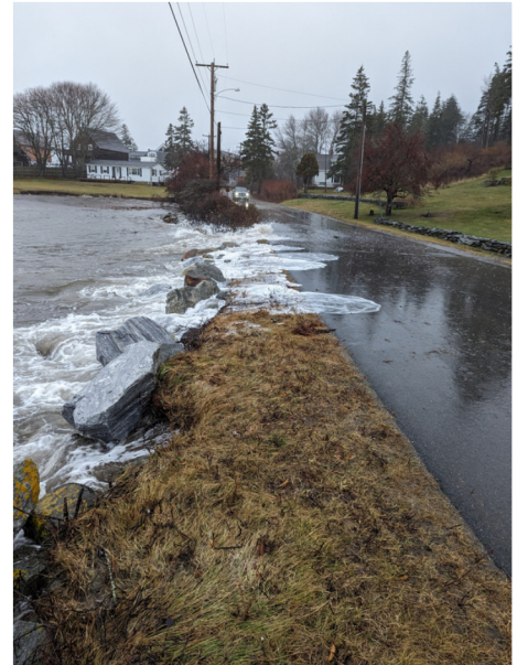
Flooding at Factory Road, Port Clyde
