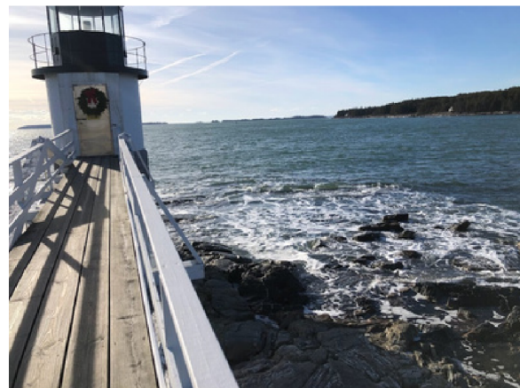
Marshall Point Lighthouse
