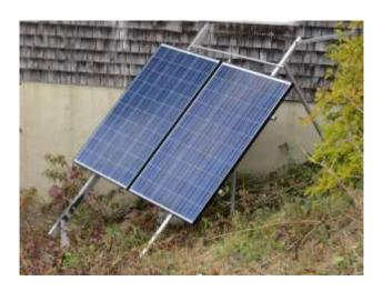
Slightly larger in size than their predecessors (above) but far more powerful, these 250-watt panels each have a small 12-VDC-to-110-AC inverter and are part of a 1.5 kW grid-tie system that provides daytime power to a year-round home. Electric bills rarely exceed \$13 thanks to conservation, Energy Star appliances, wood heat, and propane.
