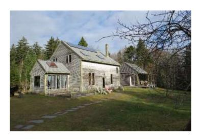
In 2002, the owners of Green Bean Catering bought 9 PV panels from Talmage Engineering for this completely off-grid system. It has 16 deep-cycle marine batteries and a back-up generator for winter. The two refrigerators are super-insulated with the motors on top. The ranges in the house and shop kitchen run on propane. Power conditioning installed by SolarWinds NorthernLights
