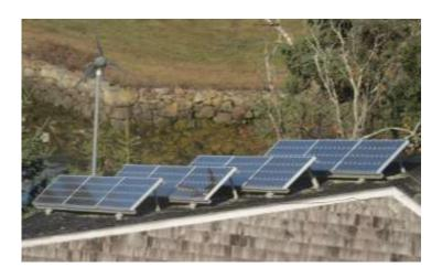
A PV system is sometimes coupled with a wind turbine for power at night. The turbine may be connected directly to batteries or an inverter. These 75-watt panels supply energy to the house and feed unused power into the grid. The panels on this page were mounted by the owner.
