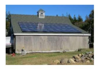
Before Central Monhegan Power was created, PV systems had begun to replace the forty noisy generators that rumbled throughout the rustic village. Today, the power company's two oil-run turbines are supplemented by a 40-panel solar array with a 10 KW industrial inverter contributing 3% of CMP's customers' power. Meanwhile, many island cottages continue to get 100% of their electricity from the sun.
